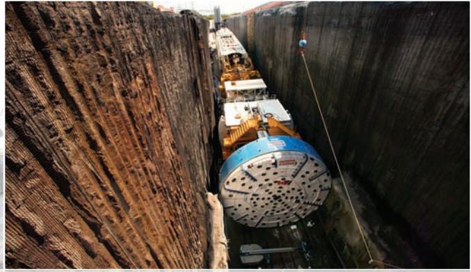
Figure 6.13 Modern tunnel-boring machines allow tunnels to be dug much faster than in the past.
