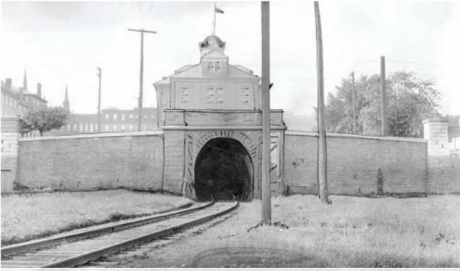
Figure 6.12 The Brockville Tunnel, Canada's first railway tunnel, took more than six years to construct.
