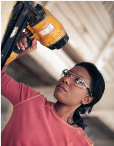
Figure 9.10(a) A pneumatic nail gun uses compressed air to drive nails into wood.
